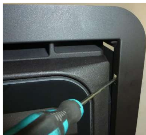
Figure No.13 - How to bend the tabs
