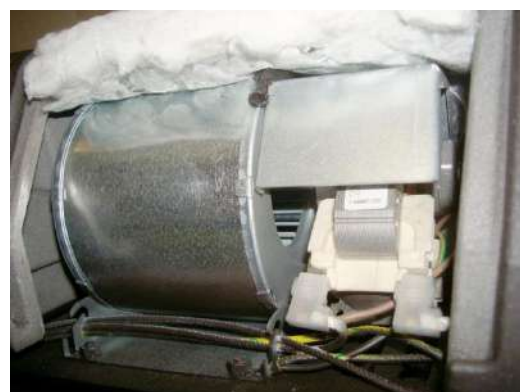
Figure No.30 - Access to fans
