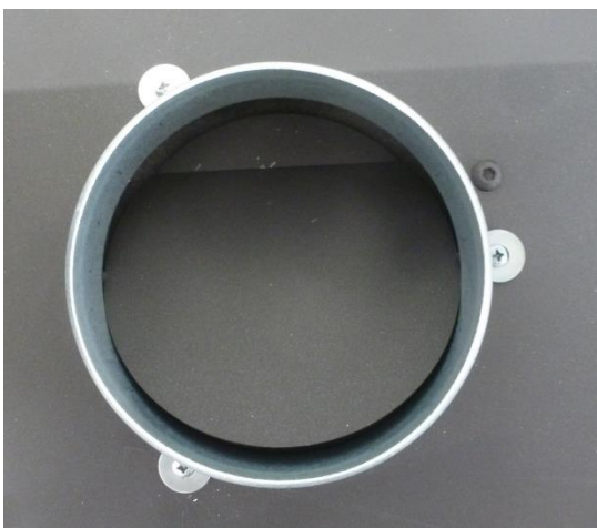
Figure No.8 - Correctly screwed nozzle at the 3 points with the washers
